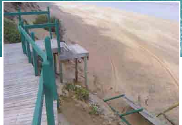
The tides rose up to the boardwalk leading down to the sea. The lower steps onto the beach and a section of the walkway were washed away.
